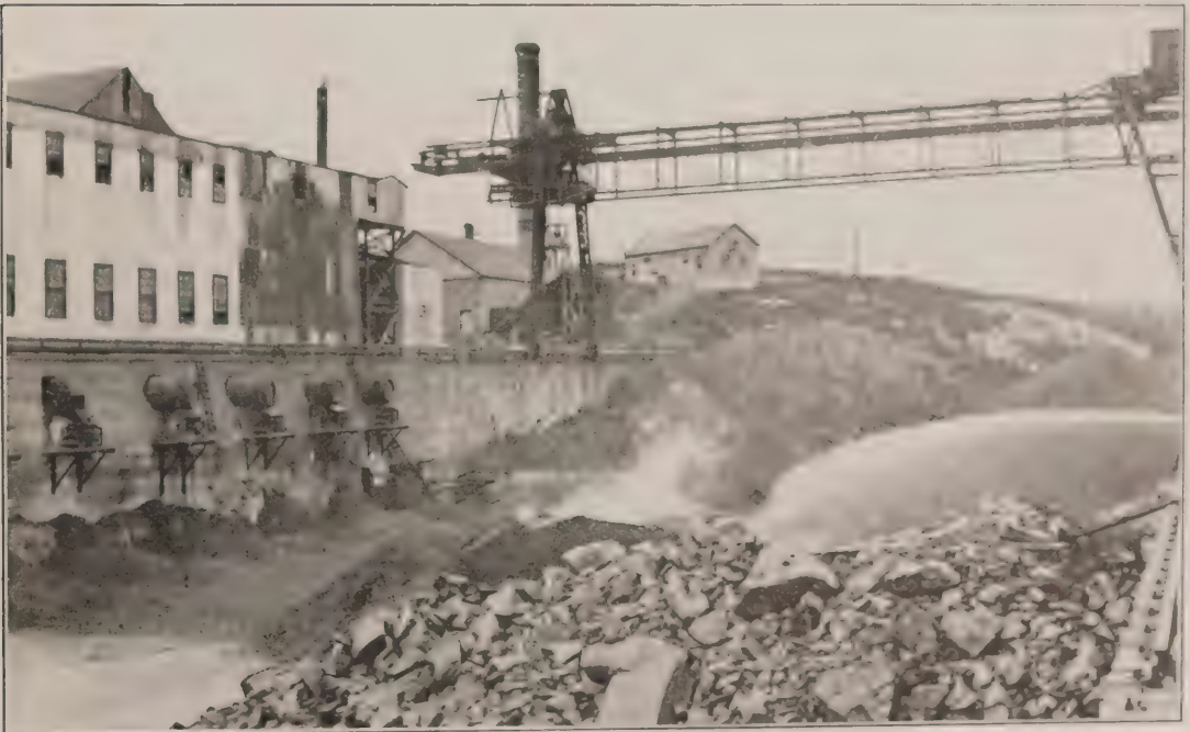
Magpie mine: discharge end of cooling tube.
